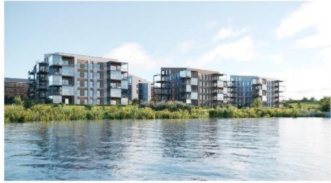
Verket Atrium block K, L, M
