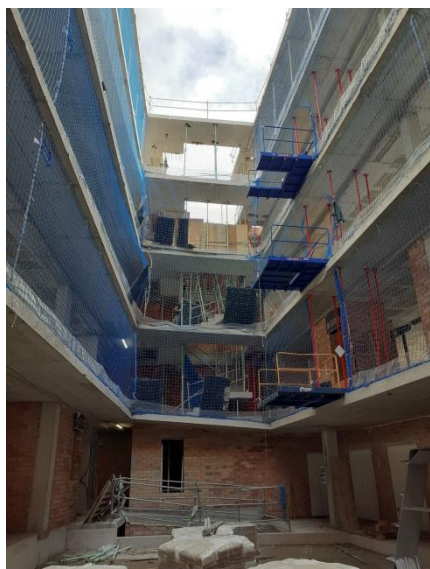
Figure 5. The construction site (March 2023)
