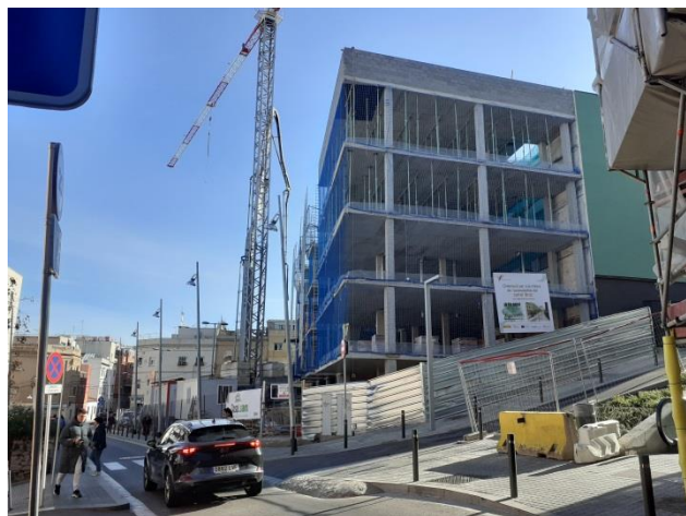
Figure 4. The construction site (March 2023)
