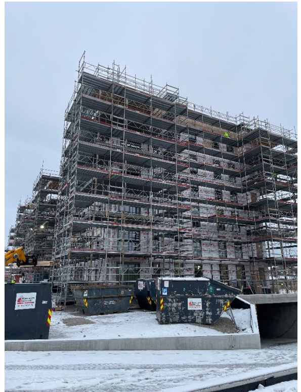
Figure 5 Photo from the construction site, January 2023
