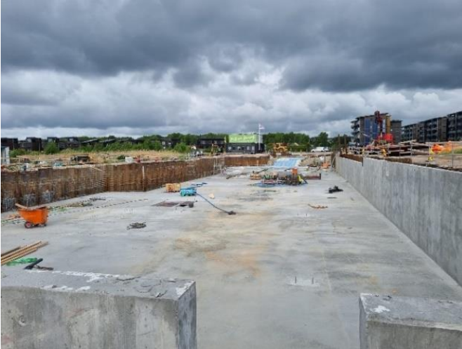
Figure 4 Photo from the construction site, June 2022
