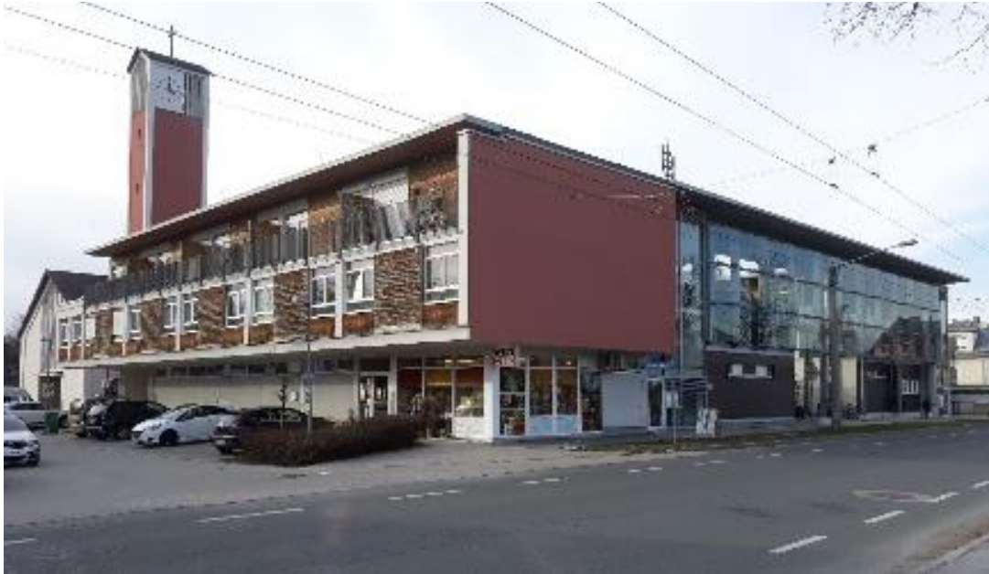
Figure 22 Demonstration project - Berchtesgadner Straße 70-72 in Salzburg, Austria. Continental Climate Demonstration Project.
