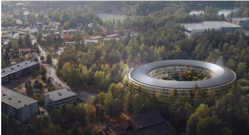
Figure 33 Design visualisation of the OEN building – initial planned subarctic climate demonstration project
